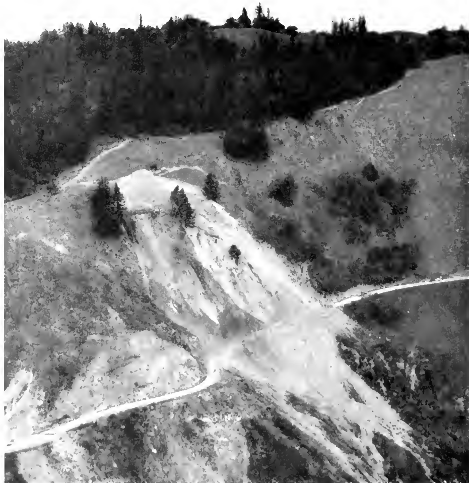
Graphic aerial photo showing extent of slide which closed Sign Route 1 between Jenner and Fort Ross
